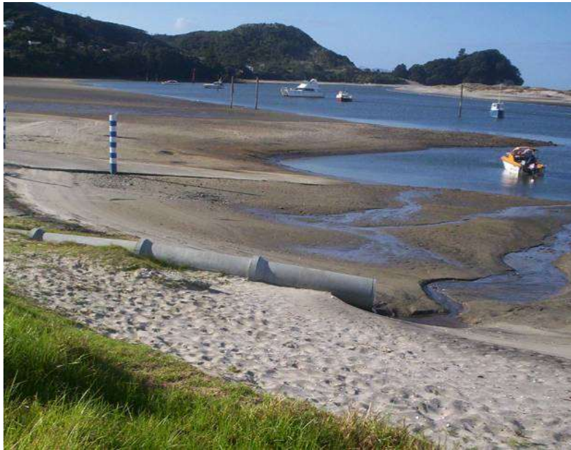
Figure 5-13: Coastal outfall, Mangawhai
