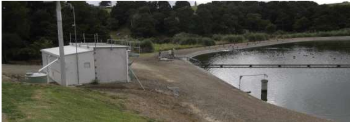
Figure 3-19: Maungaturoto WWTP oxidation pond and membrane building
