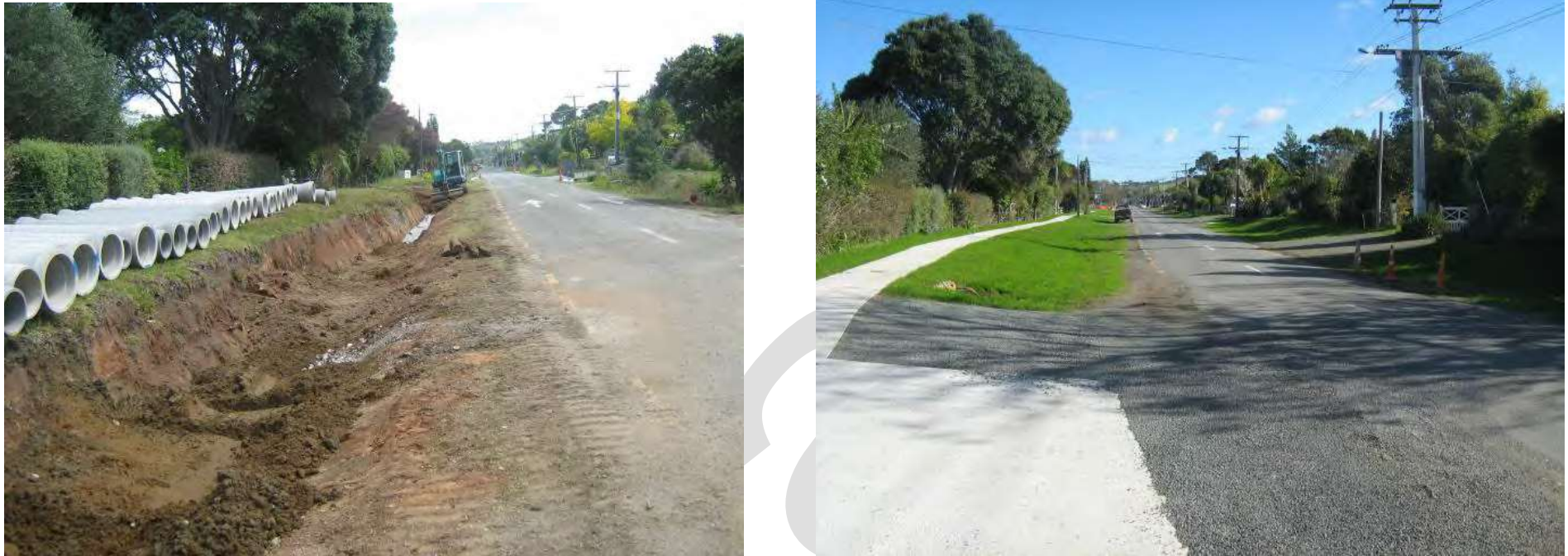
Figure 5-12: Moir Street before and after
