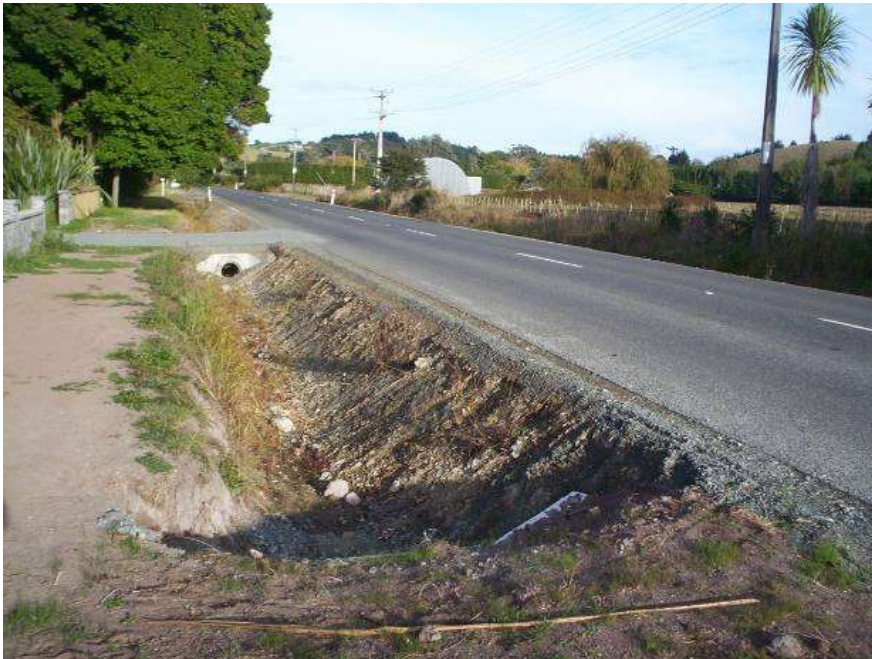
Figure 5-14: Open drains in Kaipara district
